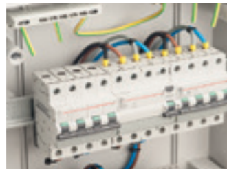
Ready to install the terminal blocks for neutral and earth connection
