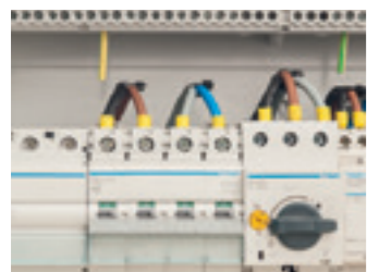
Wide space for the cabling
