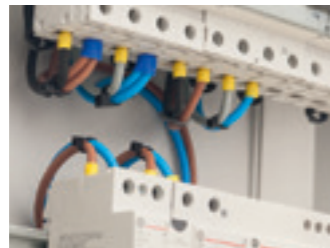
Wide space for the cabling
