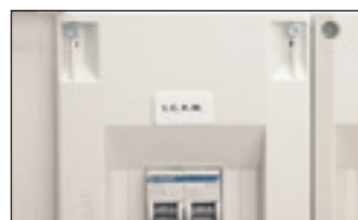
Possibility of adapting a main power breaker switch.
