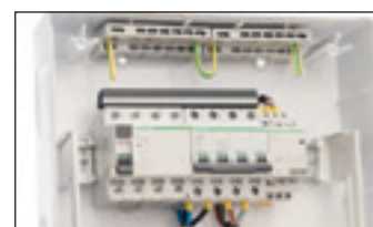
Wide space for the cabling.
